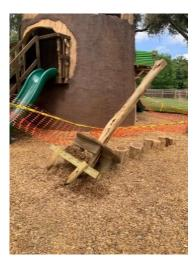
The slide exit chute has NO footing at all.
