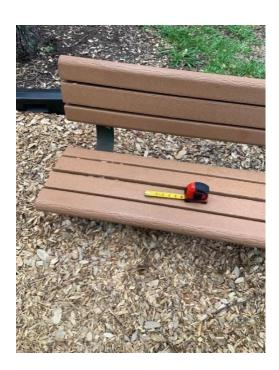
Several areas have sharp edges and non-compliant CPSC 3.4. Loose screws, 45° cut boards, edge, wood trim, 90° cut edge, not rounded.
