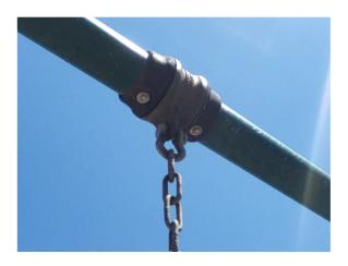
Compliant 6.7.2. Swing hangers are spaced wider than seats, not less than 20. (ASTM 8.6.1.5)
